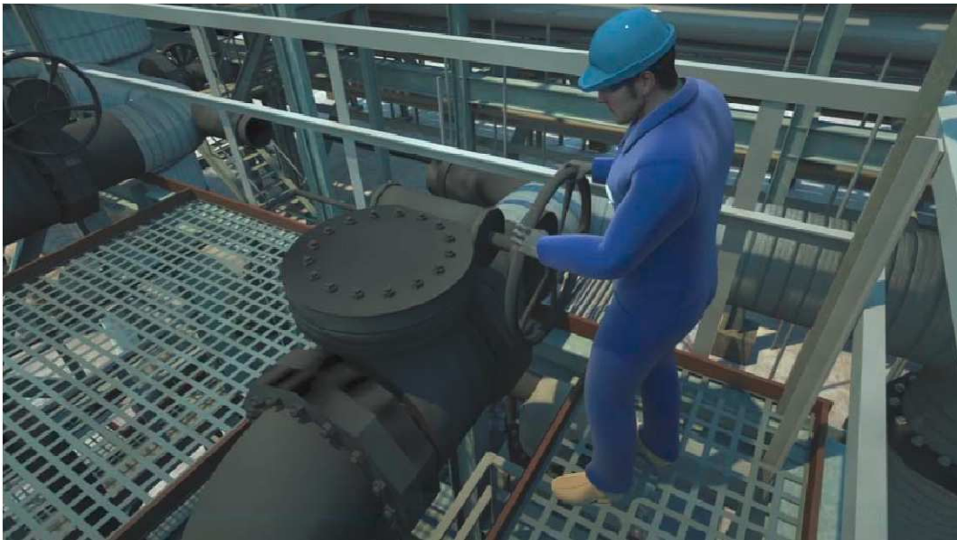
Figure 4: CSB Animation of Operator Opening a Long-Winded Valve on the Night of Incident
